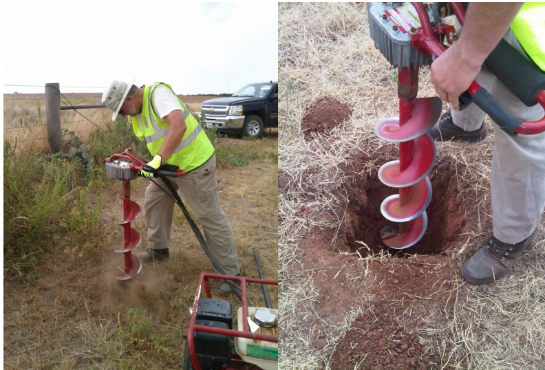
Post-hole installation using a motorised hand auger
